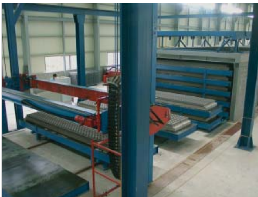
Removing and stacking the finished products
